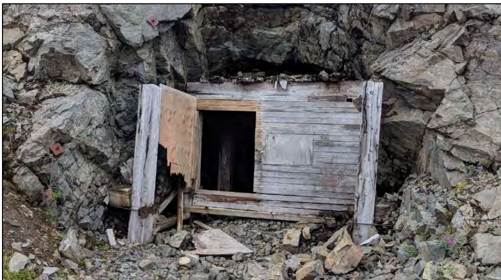
FIGURE 6.3 PORTAL OF THE DOC ZONE ADIT ACCESSING THE Q17 VEIN
